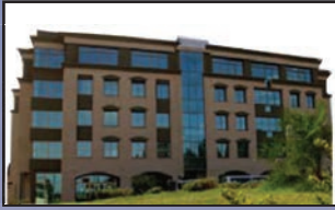
EEA Head Office Building
