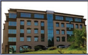
EEA Head Office Building
