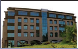
EEA Head Office Building
